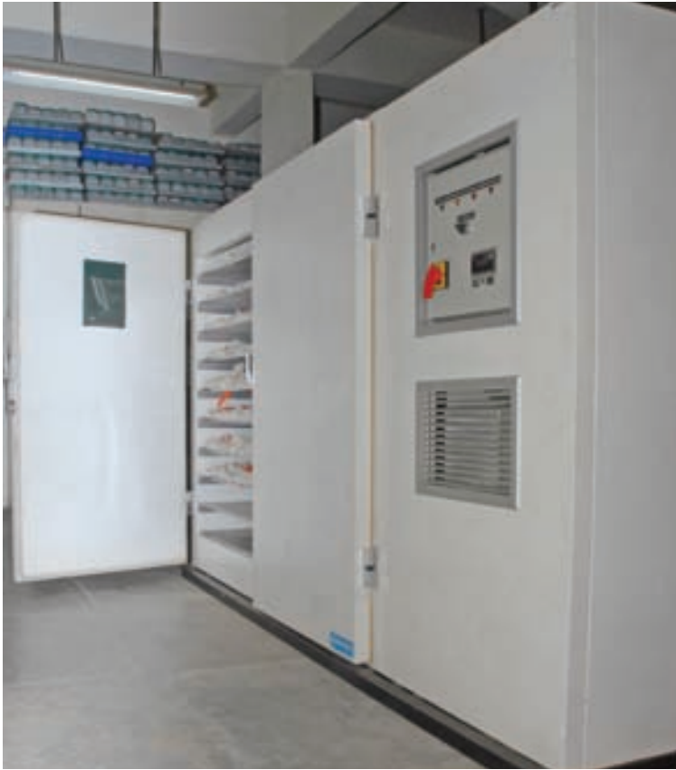
Figure 4C.1.1. Seed-drying cabinet at ICRISAT genebank.
